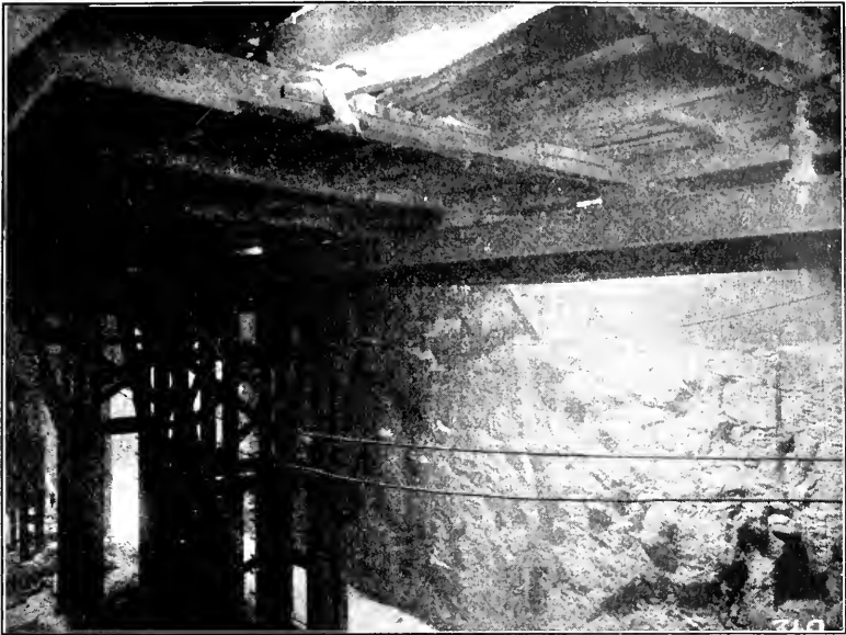
FIG. 5.—A LONG-FACE SPAN, SHOWING TOWERS, CONTINUOUS BEAMS, AND STEEL NEEDLES.
